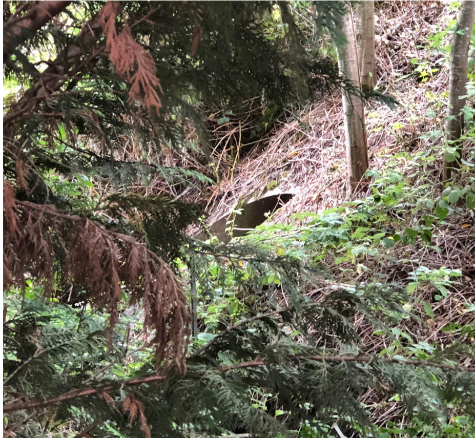
Image⑧: After flow travels under Intersate 5, flow is discharged from 54" pipe into a protected wetland.
