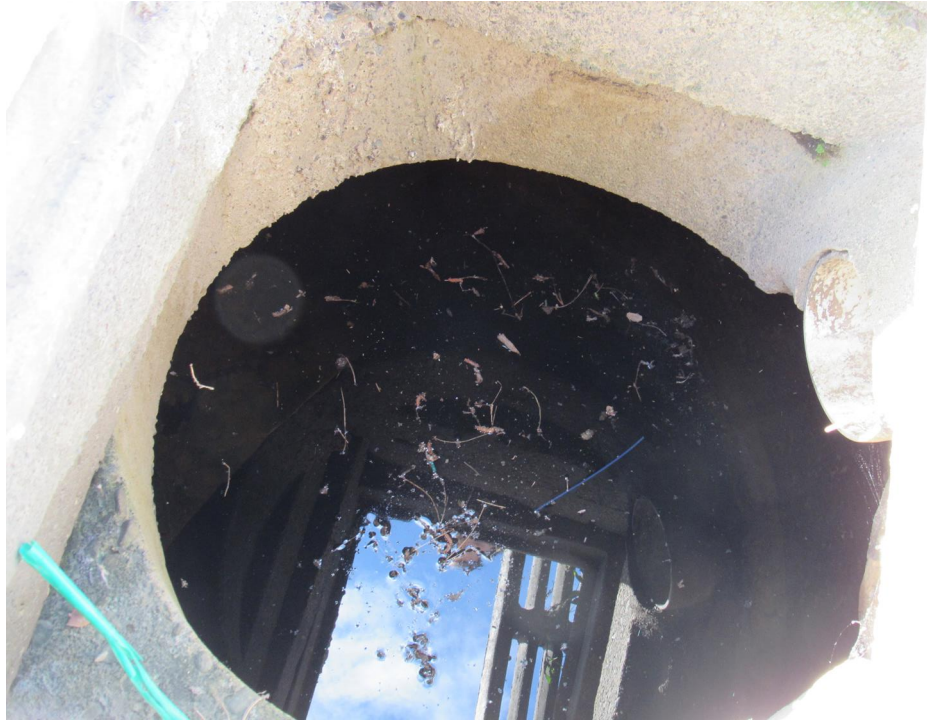
Image⑨: Flow enters another catch basin (left submerged pipe) and is redirected southeast in submerged pipe (right).
